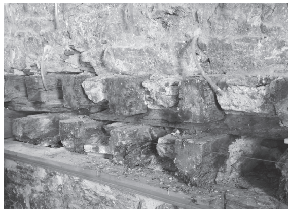
Fig. 1. Venetian part of the Bailo House. Southern wall with ends of the first floor beams exposed. Dating results: AD 1327–28.
