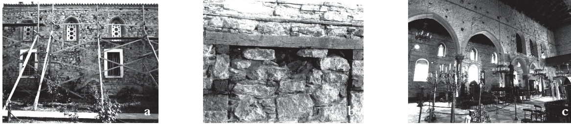
Fig. 12. (a) The north flank wall after the conservators had stripped off the plaster. The suppressed window is in the middle. (b) A typical Turkish-style lintel and transverse beams. (c) The south flank wall from the interior with the blocked window behind the candelabra. Before the nineteenth-century earthquakes the nave arcade, where now the rectangular windows are above the west gallery, would have continued on one more intercolumniation to the columns which abut the west wall on the exterior and then most likely one more interval beyond.
