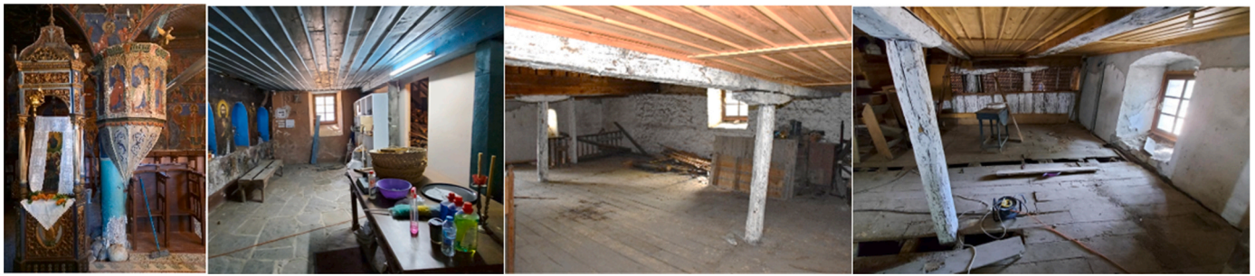
Fig. 4. The timber columns in the nave and on the ground and upper floors of the narthex.
