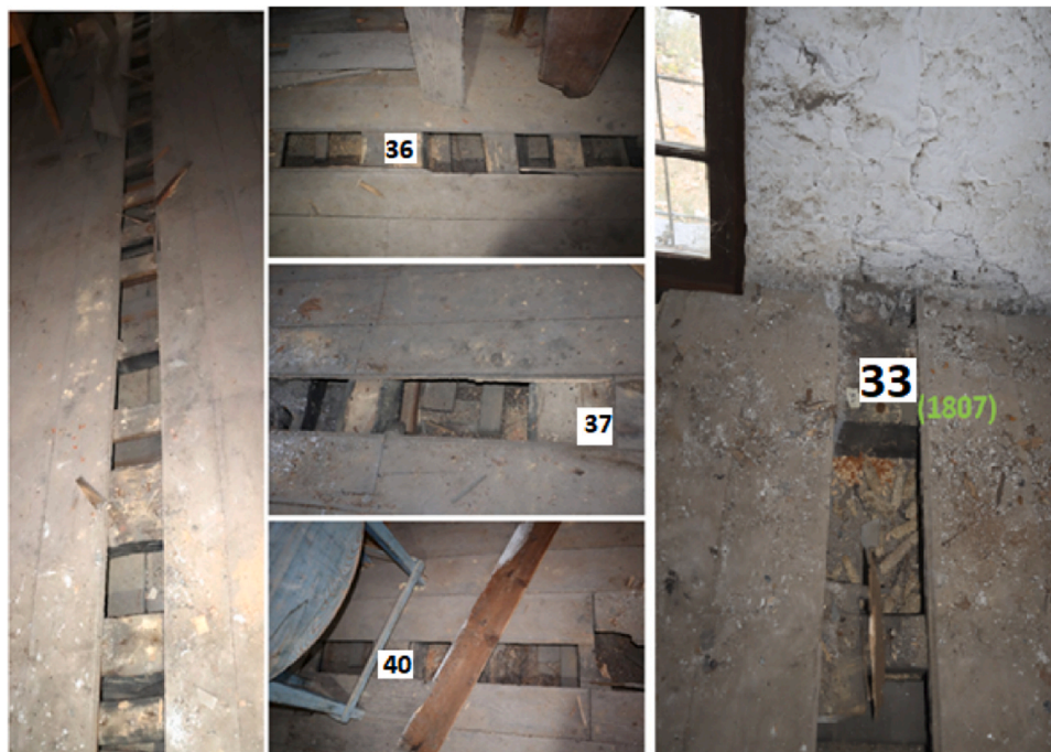
Fig. 11. Revealed beams from the floor of the narthex (Samples 33, 36–37, 40).
