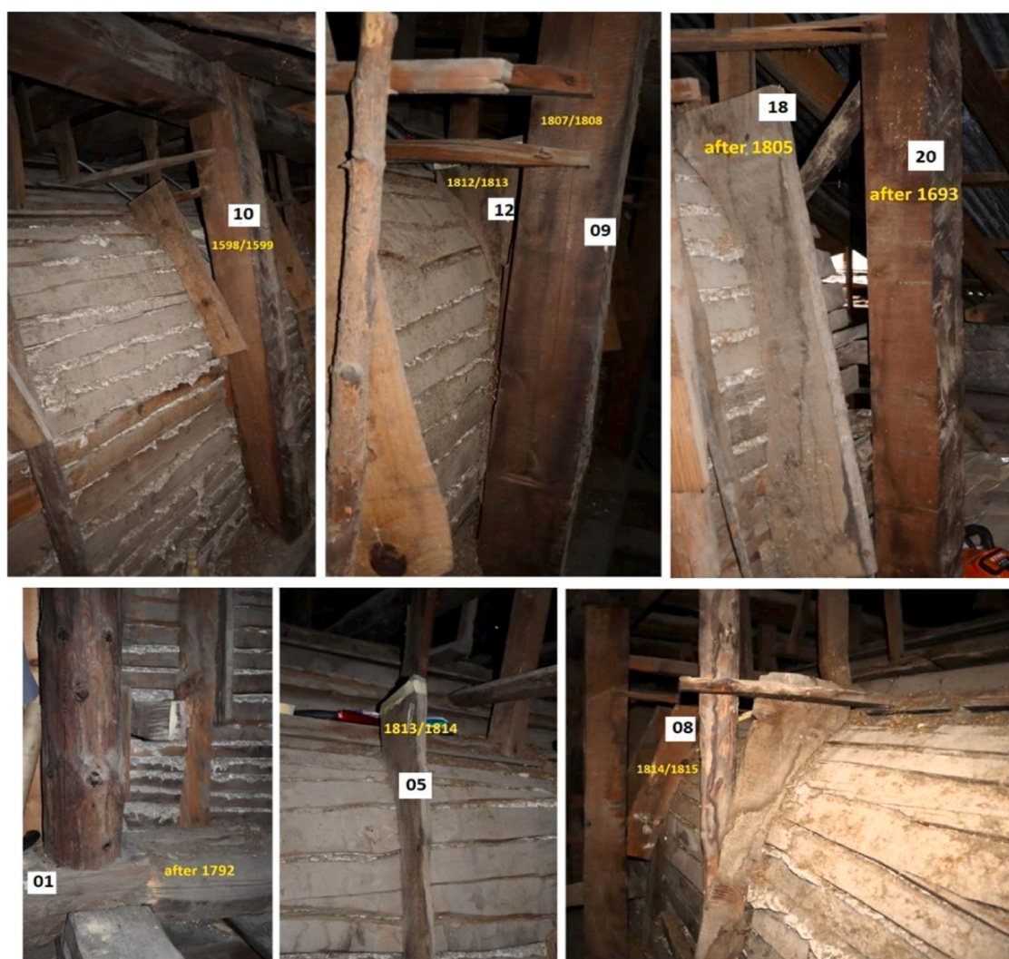
Fig. 8. Dated roof posts and curved elements of the load-bearing timbers of the vaulted central ceiling.
