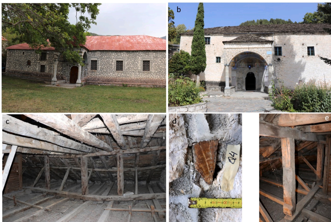
Fig. 6. Churches under restoration on the slopes of Mt. Smolikas where dendroarchaeology was applied: (a) the Pades church of the Assumption of Virgin Mary, (b) the Palaioseli church of Agia Paraskevi, (c) The roof construction in the Palaioseli church, (d) A timber inside the masonry wall made of deciduous oak in the Pades church, (e) The re-used timber from the 15th century CE in Palaioseli's roof construction.
